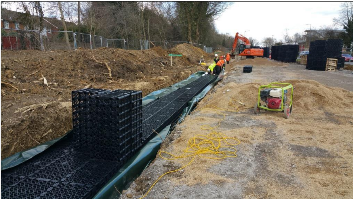
Underground drainage tanks being laid during works at the Stocklake site
