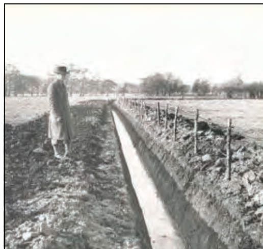
Photograph of land agent inspecting a drainage scheme at Denham (phDenham104)
